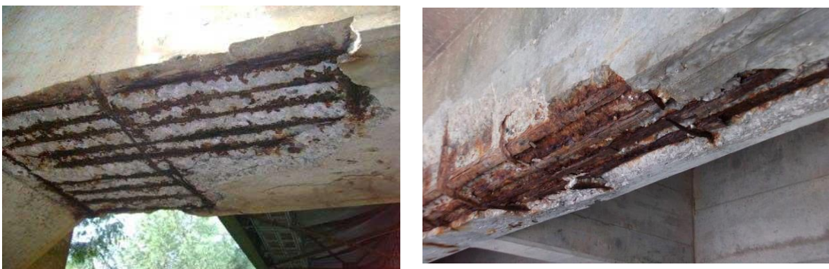
Fig.5.11 Corrosion of RCC structure
