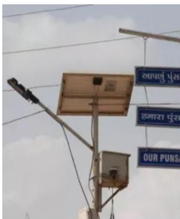
Fig. 1.29 Solar light &amp; CCTV
